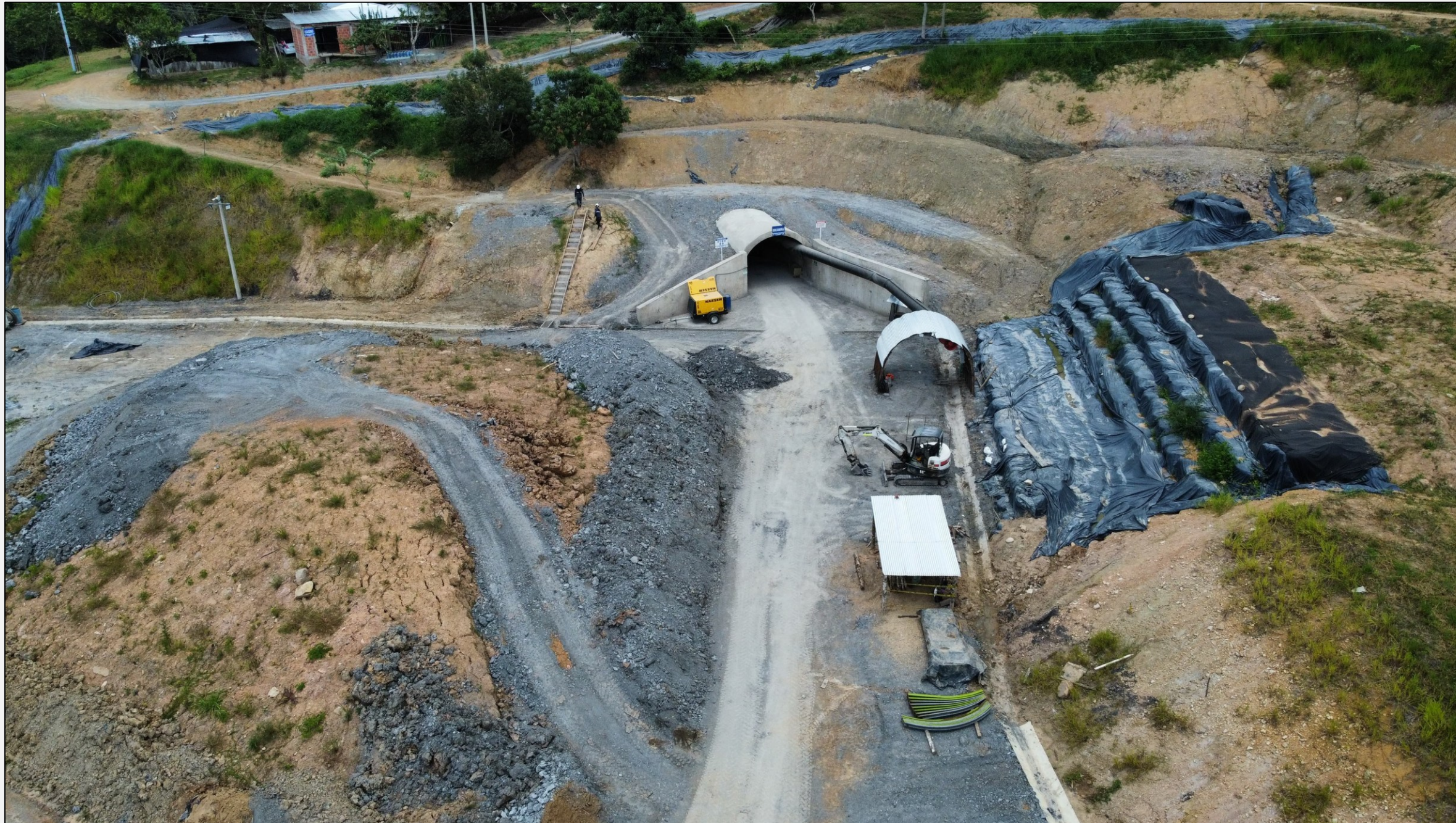
Portal Construction finalized March, 2025
