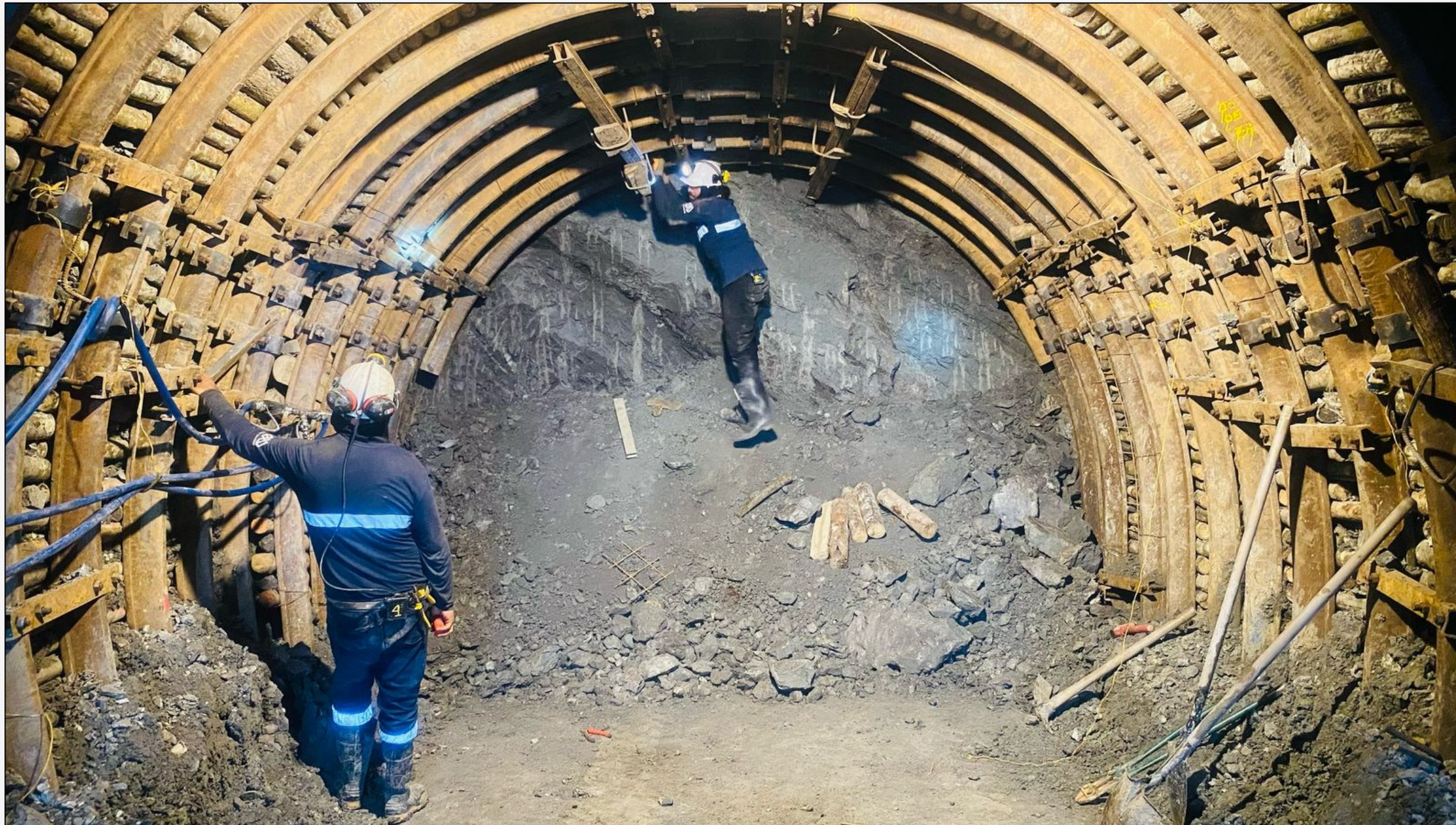
Underground decline development
