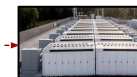
LFP Batteries
